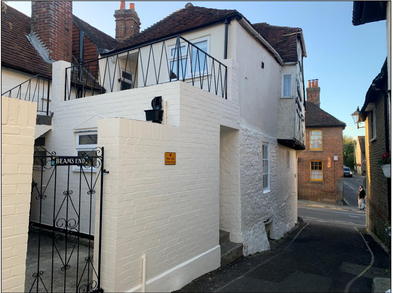
ENTRANCE TO MAISONETTE IN DUCK LANE (BEAM'S END)
