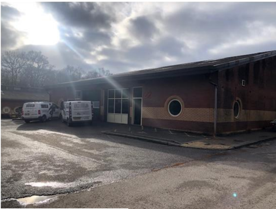
Image of Unit 22 during refurbishment
