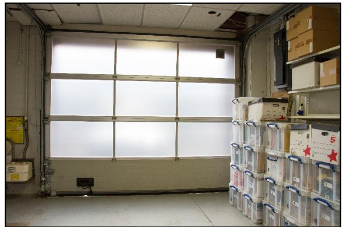
Loading & Storage Area
