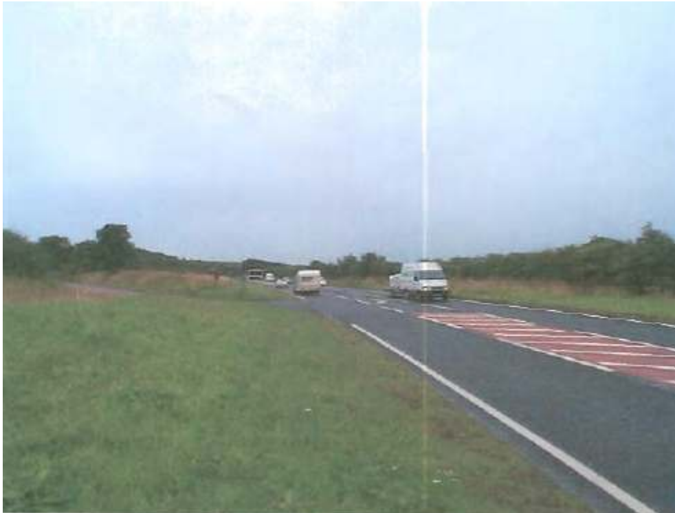
POINT D – LOOKING SOUTH
